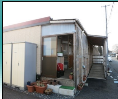
Fig.4 Temporary housing for evacuees. Slope was build additionally for a wheel chair user.
