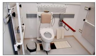
Figure 2. The toilet with adjustable devices
