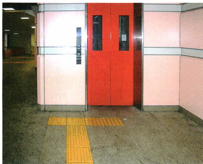
Figure 2-32: Example of leading to an elevator
