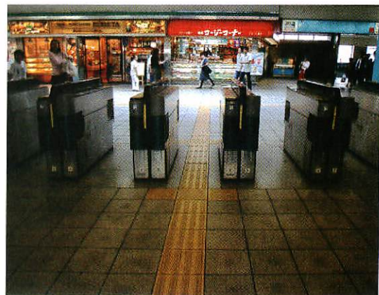
Figure 2-26: Example of installation at a ticket gate
