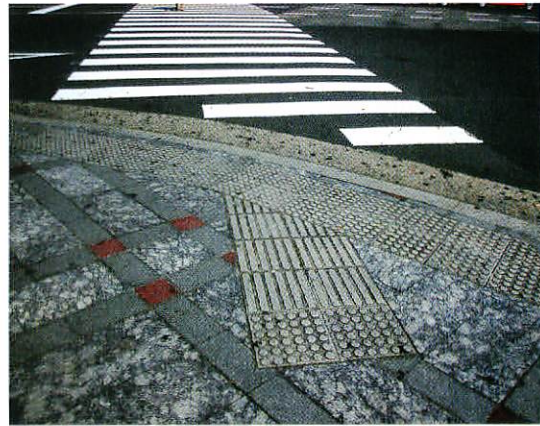
Figure 2-5: Example of an adjoining surface with low visual contrast, which makes it difficult for visual impaired people to detect tactile ground indicators
